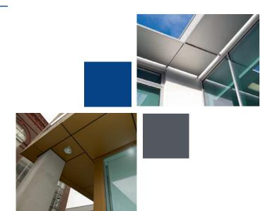
Fascias and Soffits are generally fabricated from 3mm aluminium and can be produced to your exact specification \*\*
